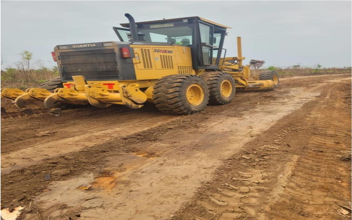
Figure 5: Reshaping of 30km of roads in the municipality
