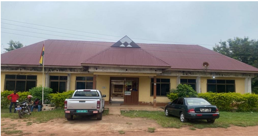
Renovation of GES office block (DACF) – Re-roofing completed
