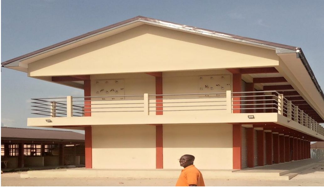
Completed 2 storey 48 unit Lockable stores and external works at Berekum Thursday Market (GSCSP)
