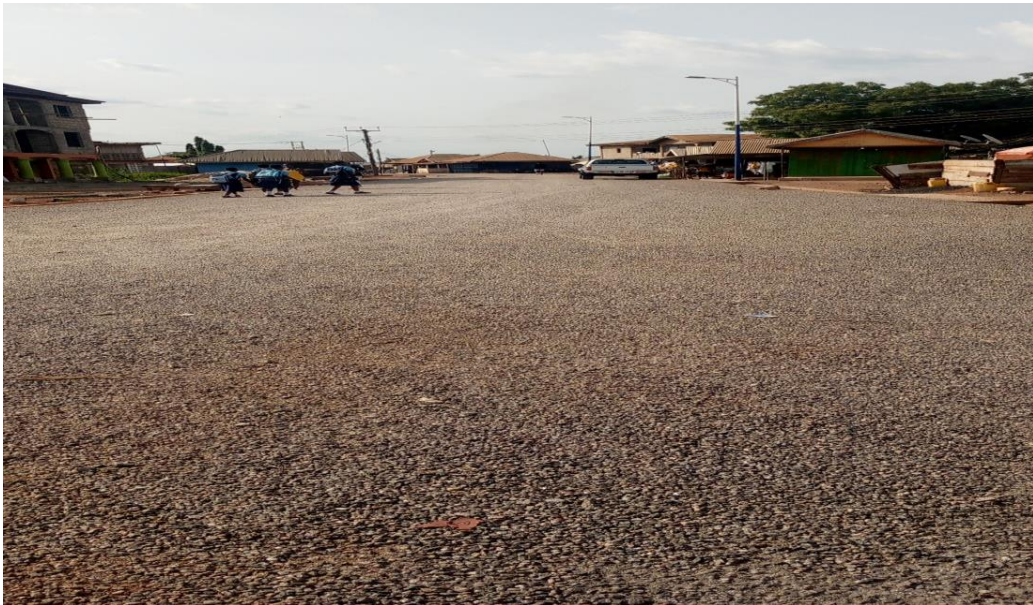
Tarred 243m road, installation of street lights, 1No. Traffic light and transformer
