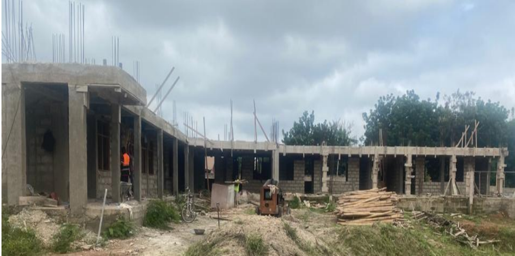
Const. of 1 storey 10-unit office complex at Berekum (DACF-RFG)
