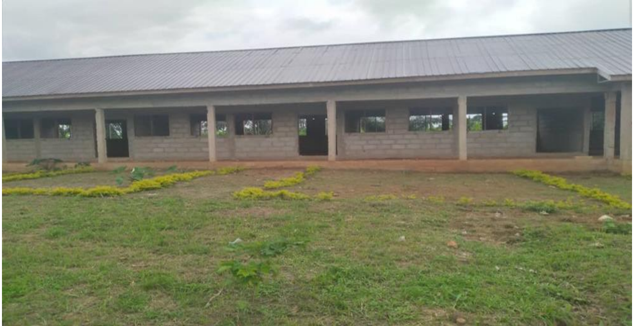
Completion of 1 No 3 Units classroom block at Norbekaw Meth JHS (On-Going)
