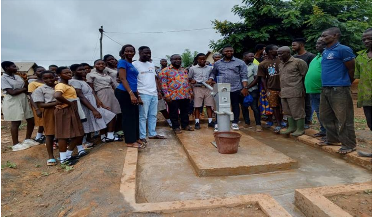
Mechanized 1No.2 Boreholes with Hand pump at Kwadoma and Pafo FUNDING: DACF
