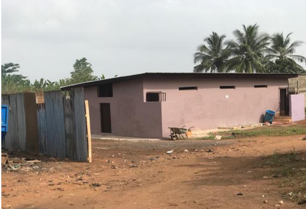
Renovated 1No. 12-Seater Aqua Privy Toilet at Kukuom FUNDING IGF
