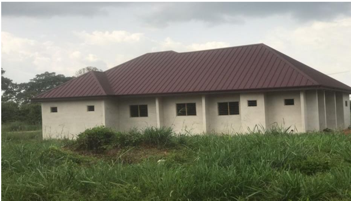
Completion of 1No. CHPS Compound at Amankwaakrom - On-Going
