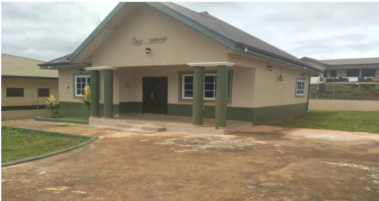
Completed 1No. 2-bedroom master's bungalow – Kukuom SHS FUNDING: Ghana Gas
