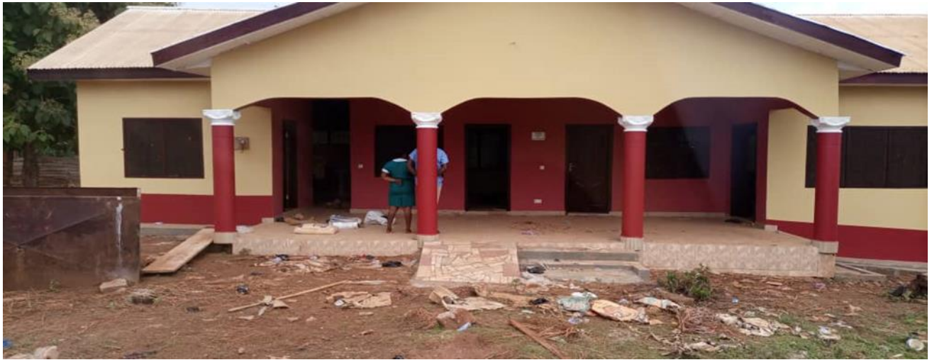
Completion of 1 No CHPS Compound – Asarekrom
