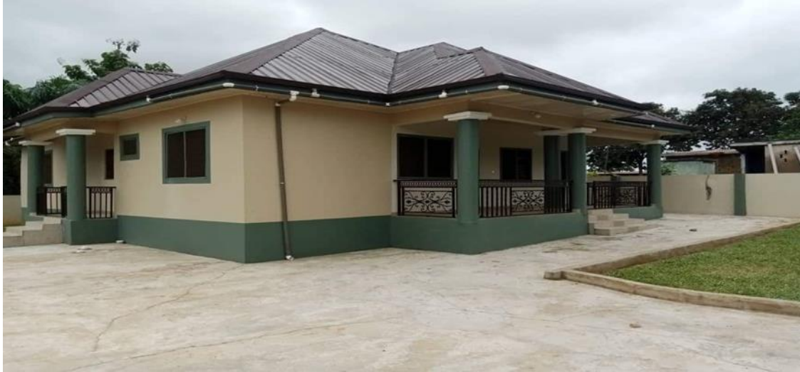
Completed 1No. 3bedroom Doctor's bungalow at Sankore FUNDING: Ghana Gas
