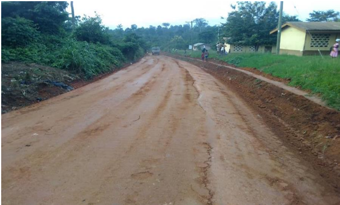
Reshaped of 8kg feeder road – Nsedua to Naketey.
