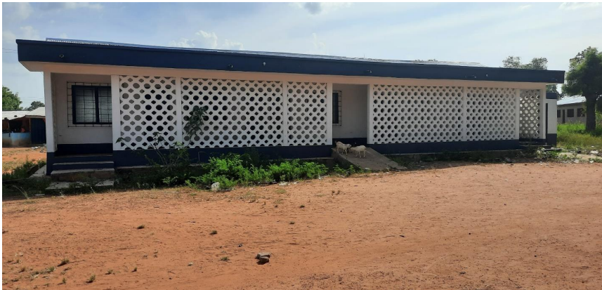
Renovated Ino. Area Council Block at Garu (DACF)
