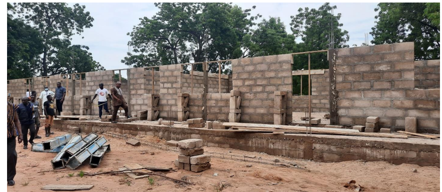
Constructed 1 no. 3-Unit Classroom Block with Ancillary Facilities at Zaa-Zua (DACF-RFG)
