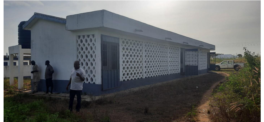
Renovated Ino. Area Council Block at Kugri (DACF)
