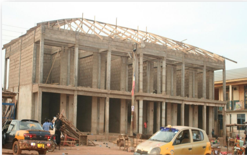
Figure 3: Construction of 1 No. 24-Unit Market Storey at Bimbilla
