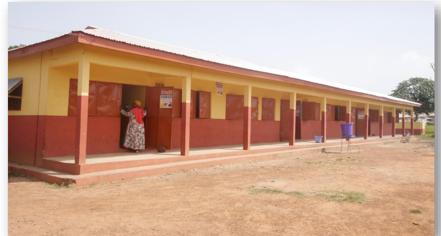
Figures 4: Constructed 1 No. 3-Unit Classroom Block at Karaga JHS
