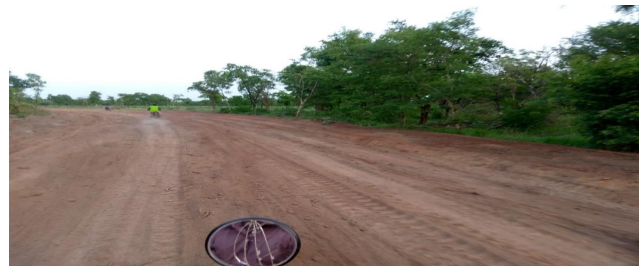
Fig.2: Simoli-Gbutugu-Yapalsi 6km Feeder Road
