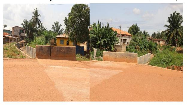
> A 0.9m Pipe Culvert/U-Drain has been constructed at Abed (Funding Source: DACF)
