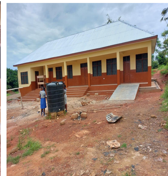
1NO. 3-UNIT CLASSROOM BLOCK AT TANOSO SDA PRIMARY SCHOOL, FUNDING: GRC
