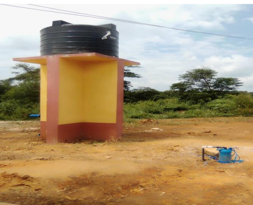
NO. MECHANIZED BOREHOLES, LOCATION: ASSEMBLY RESIDENCY ABUOM BREDI CHP COMPOUND
