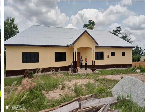
Construction of Hostel facility at Tanoso CHNTS of Health. Funding: DACF
