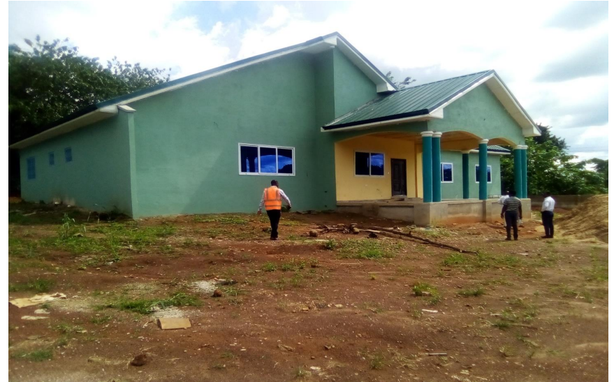
Construction of DCE's Bungalow at Hwidiem (DACF)
