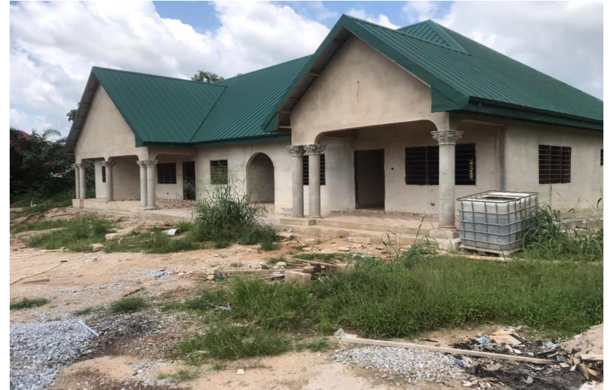
Construction of 1No. 3-Unit Teachers Accommodation at Bronikrom (DACF-RFG)
