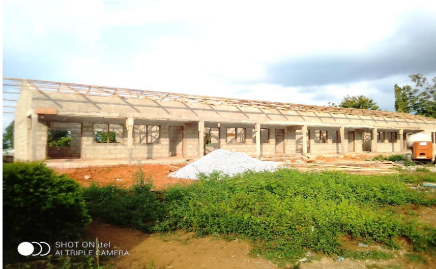
Construction of 1No. 4-Unit Classroom Block at Amanfrom (DACF-RFG)
