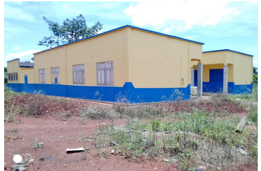
Construction of 1No. 3-Unit Classroom Block with 3 Bedroom Dormitory Accommodation at Dadiesoaba Girls Model School
