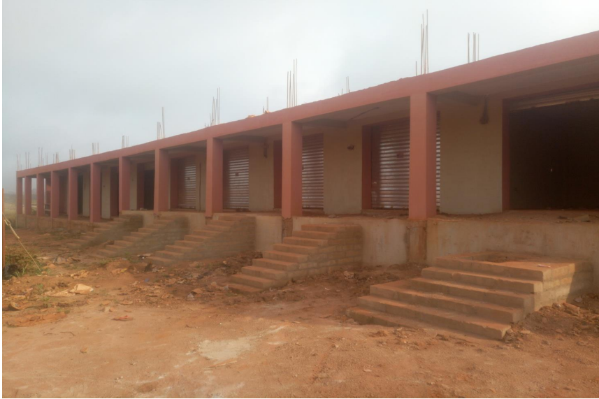
Construction of 1No. 10-Unit Lockable Market Stores at Hwidiem (DPAT)
