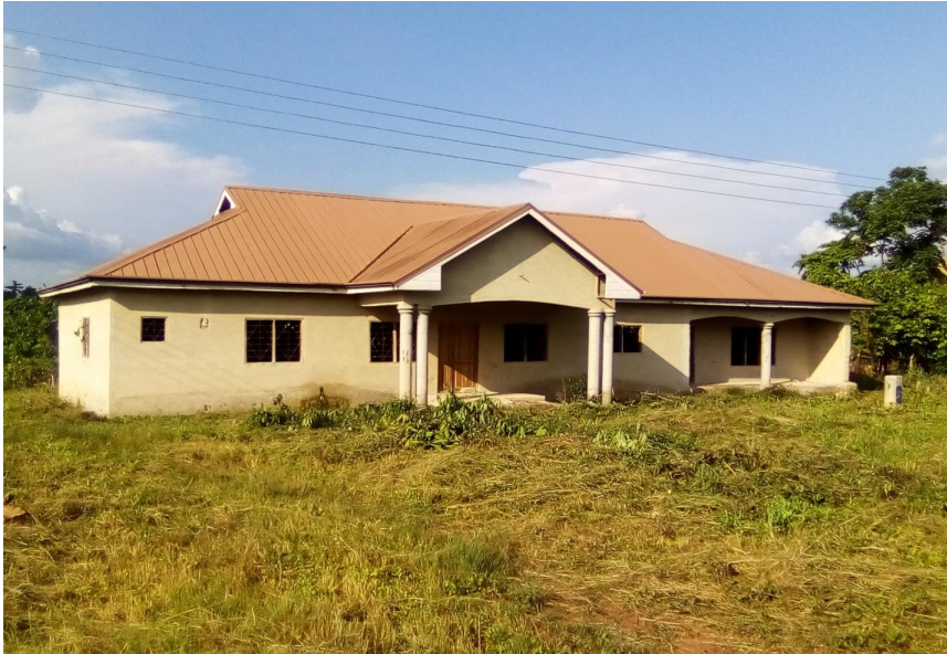
Construction of 1 No.CHPS Compound at Mehame (DA CF)
