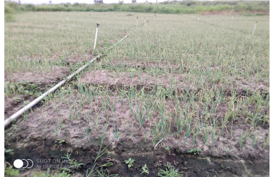
Construction of Irrigation Facility at Hwidiem (DA CF)
