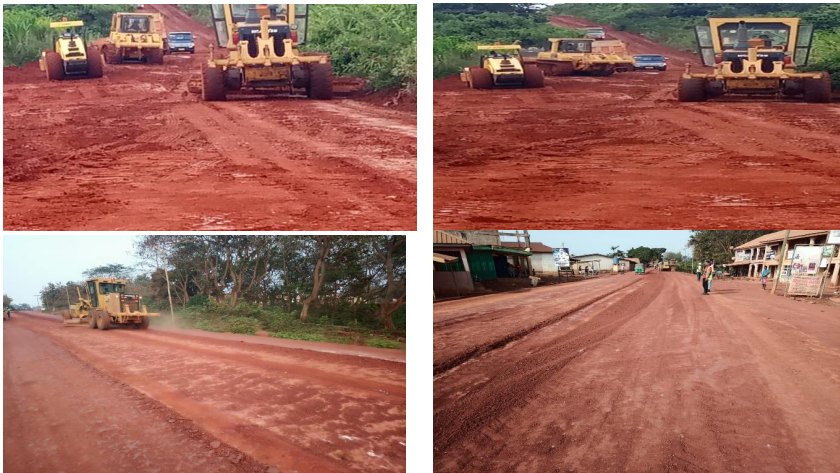
RESHAPED GAMBIA-DORMAA BARRIER ROAD
