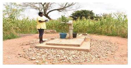
DRILLED BOREHOLE WITH HAND PUMP AT SOE ALARABISI UNDER DACF
