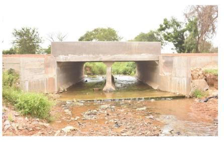
EMERGENCY CONSTRUCTION OF 2.5m x 1.5m DOUBLE BOX CULVERT WITH 0.9m U DRAINS AND APPROACH FILLING AT SOE NEW TOWN
