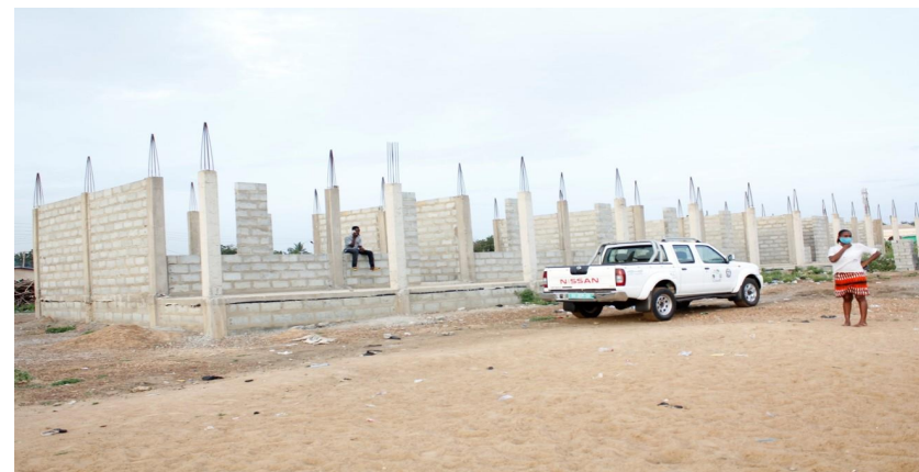
CONSTRUCTION OF 2 STOREY 6 UNIT CLASSROOMBLOCK AT HANNA (PHASE1)
