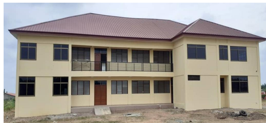
CONSTRUCTION OF 1 NO MUNICIPAL COURT AT GBETSILE
