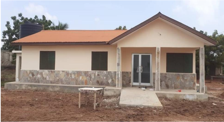
RENOVATION OF HEALTH FACILITY AT KATAMANSO
