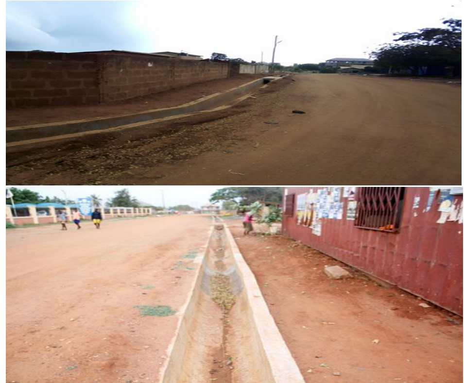
CONSTRUCTION OF 2KM METROPOLITAN, MUNICIPAL ASSEMBLY(MMA) LOCAL DRAIN IN KPONE
