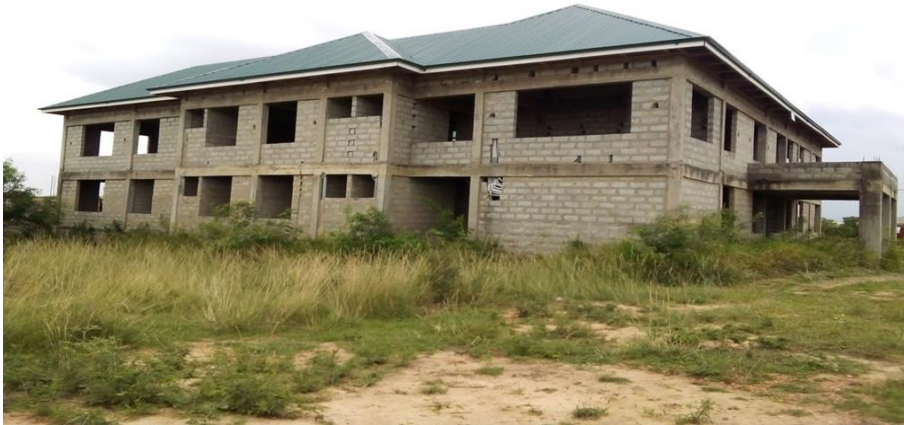
CONSTRUCTION OF 1NO 2 STOREY HEALTH FACILITY AT GBETSILE
