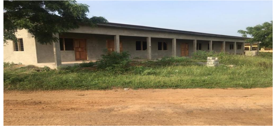
CONSTRUCTION OF 1 NO 3 UNIT CLASSROOM BLOCK AT OKUSHIBRI
