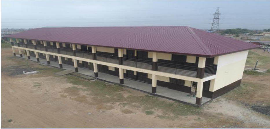
CONSTRUCTION 2 STOREY 6 UNIT CLASSROOM BLOCK AT SANTEO
