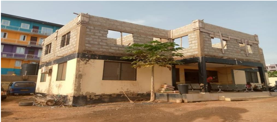
CONSTRUCTION OF 2 STOREY COMMUNITY POLICE STATION AT OYIBI
