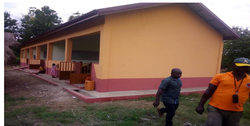
3 Unit pavilion classroom at Amule
