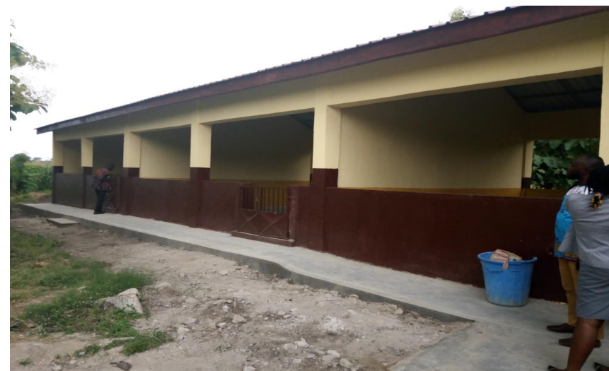
3 Unit Pavilion Classrooms at Atanve
