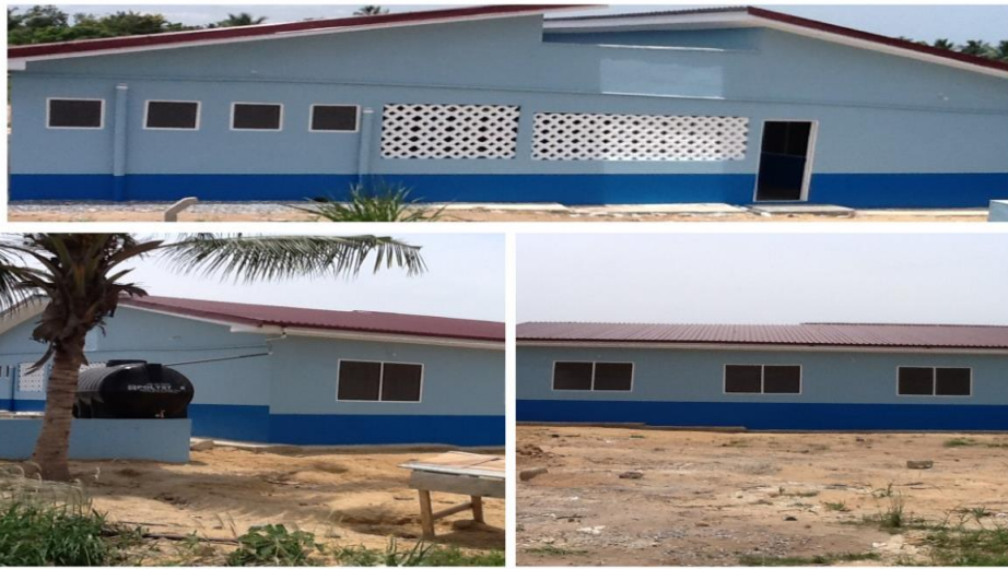
CROSS SECTIONAL VIEW OF COMPLETED HOBOR CHPS COMPOUND
