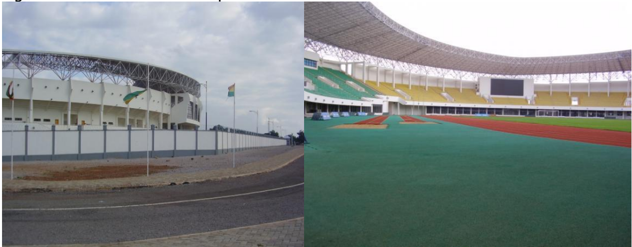
Figure 3: Picture of the New Sport Stadium
