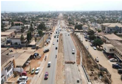
La Beach Road Completion Project
