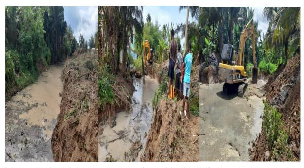
Dredged Evaley & Ayile Storm Drains 2.1km and Dredged Effia Storm Drain to a distance of 1.2km
