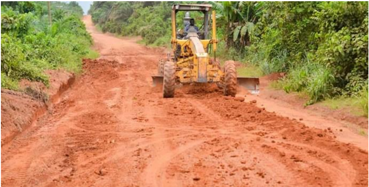
Reshaped 56.40 Km feeder roads districtwide.
