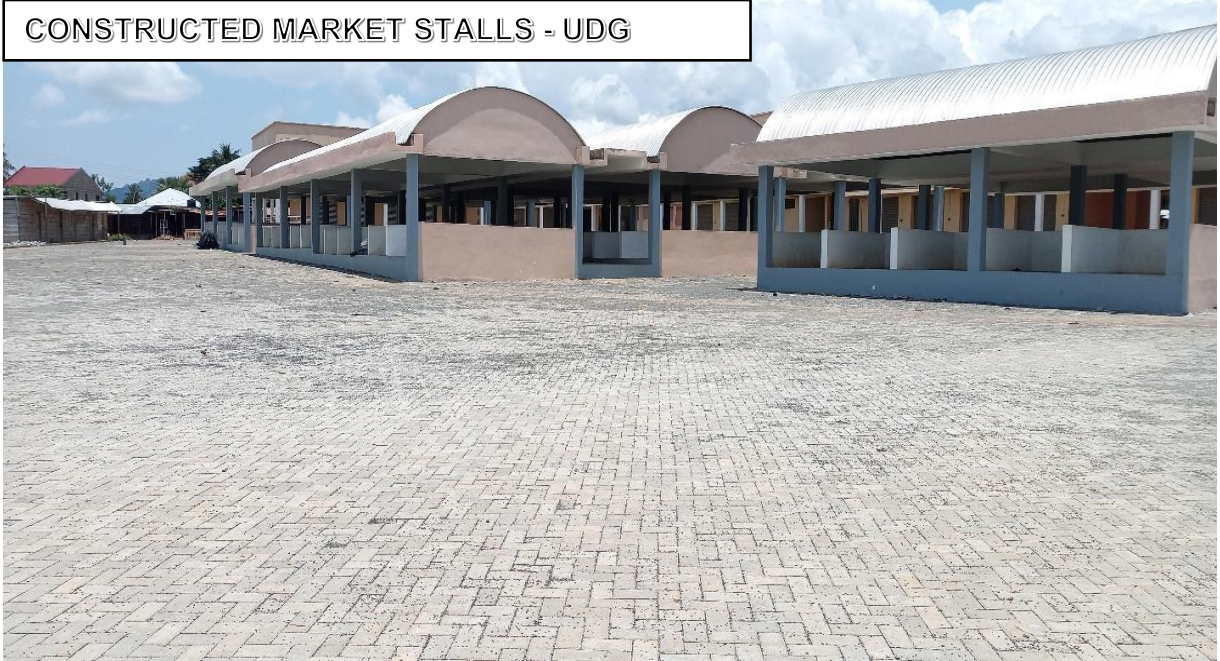
CONSTRUCTED MARKET STALLS - UDG
