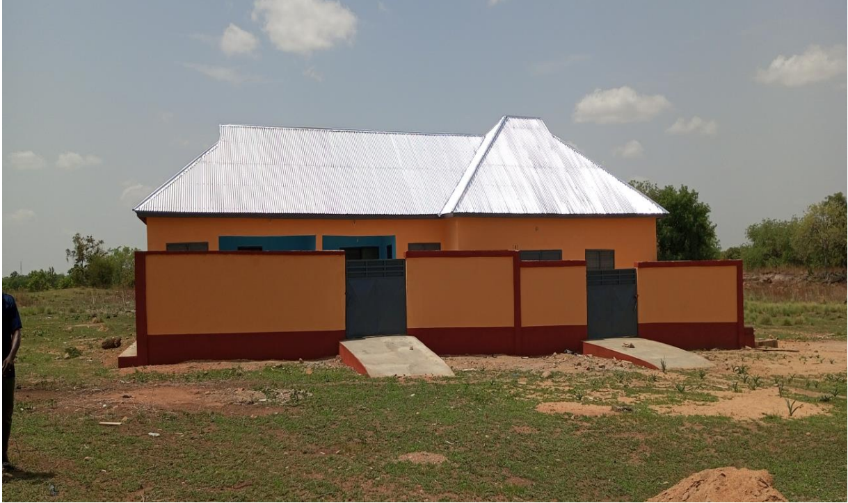
Figure 2. Constructed and furnished 1No. CHPS compound at Basissan
