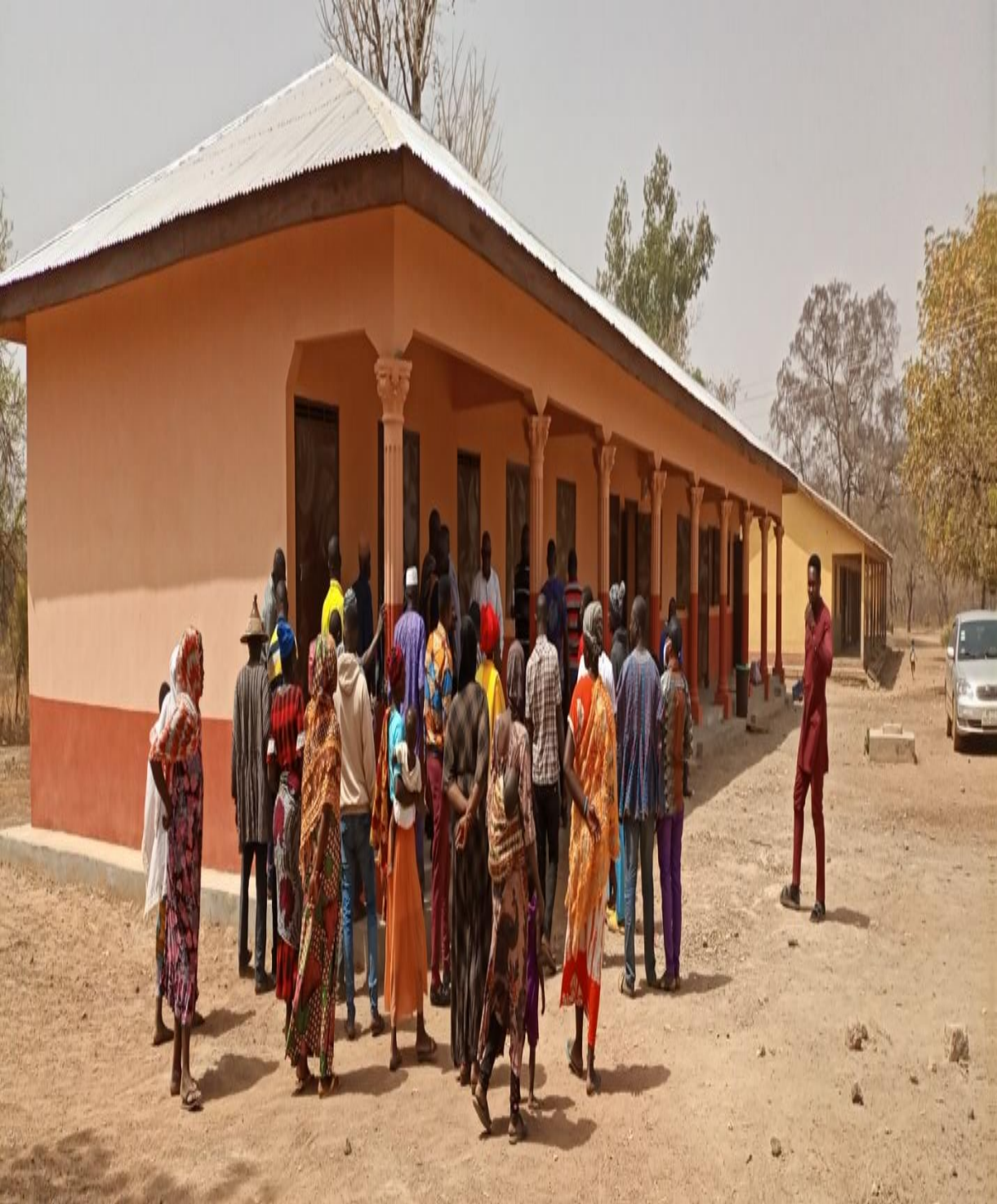
Figure 1. Constructed and furnished 1No 3-unit classroom block with office, store and staff common room at Dimajan Primary
