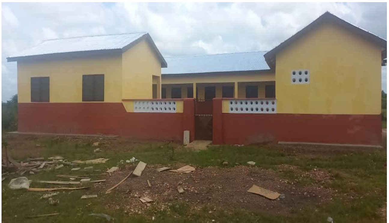
Figure 2: Constructed 2-unit KG Block at Methorbuo.
