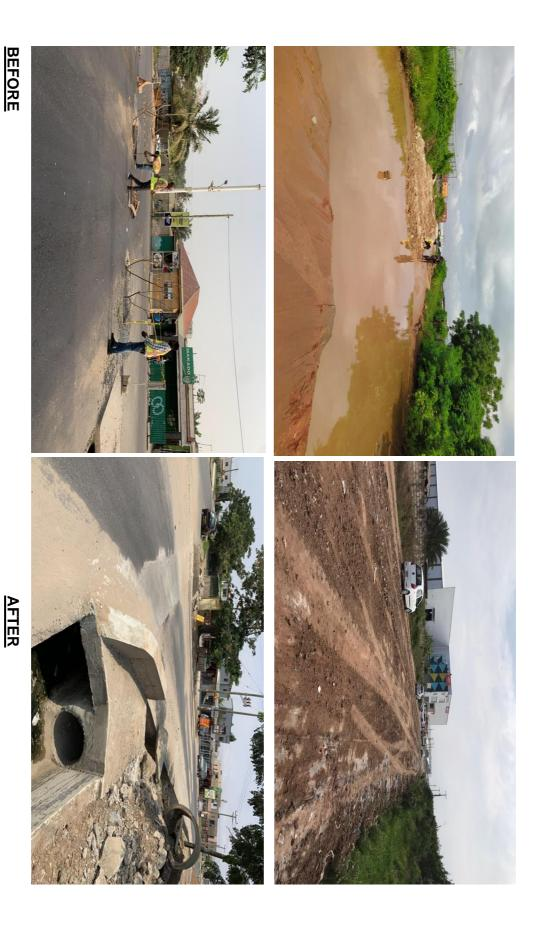
**JOTAFA** CONSTRUCTED 900MM AND 1200MM PIPE CULVERTS AND APPROACH FILLING ON MLIA ROAD AND LAY BY AT
