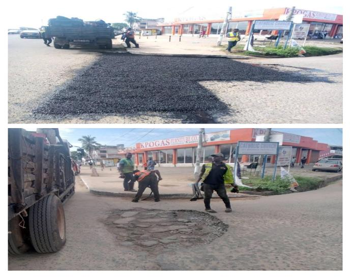
FIGURE 7 POTHOLE PATCHING WITHIN THE MUNICIPALITY
