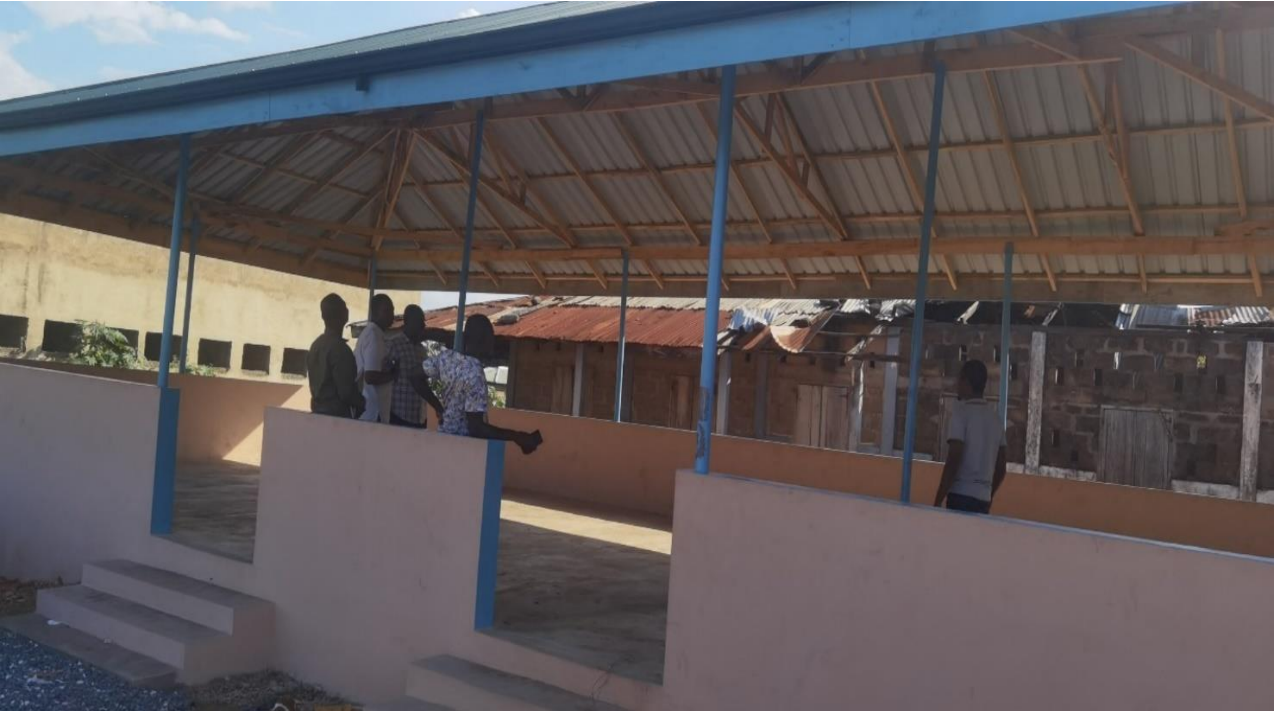
Constructed of 1no market pavilion at Kpong
