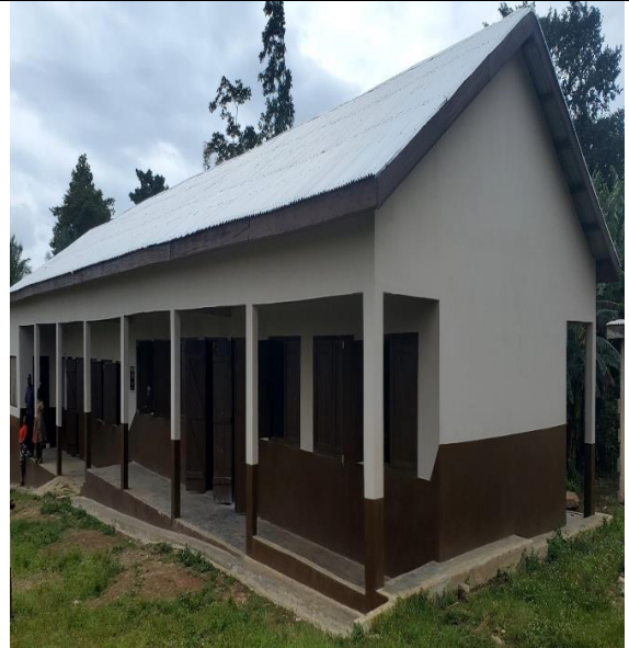
Completed 1No. 3-Unit Classroom Block, Urinal, KVIP and Office at Kwahu Tafo.
