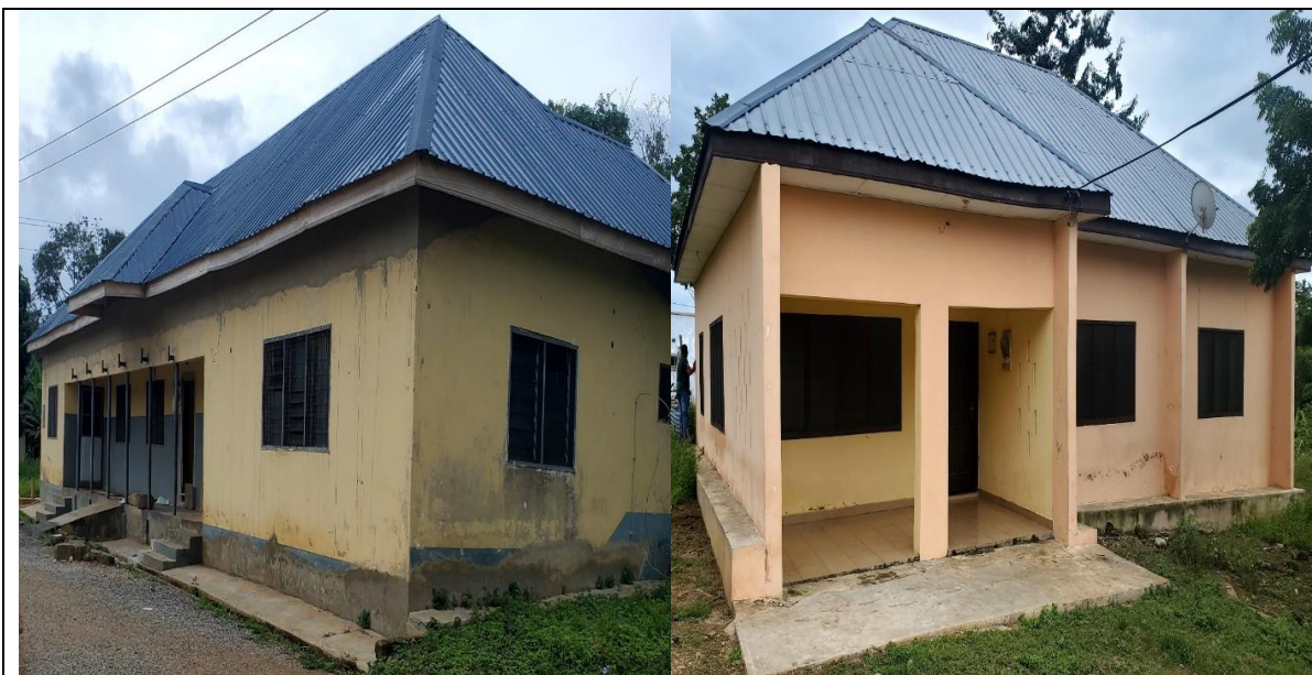
Rehabilitation of Bokuruwa CHPS compound & Nurses' Quarters (65% Completion)
