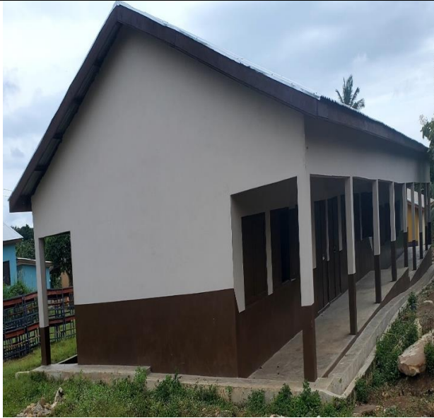
Completed 1No. 3-Unit Classroom Block, Urinal, KVIP and Office at Kwahu Tafo.
