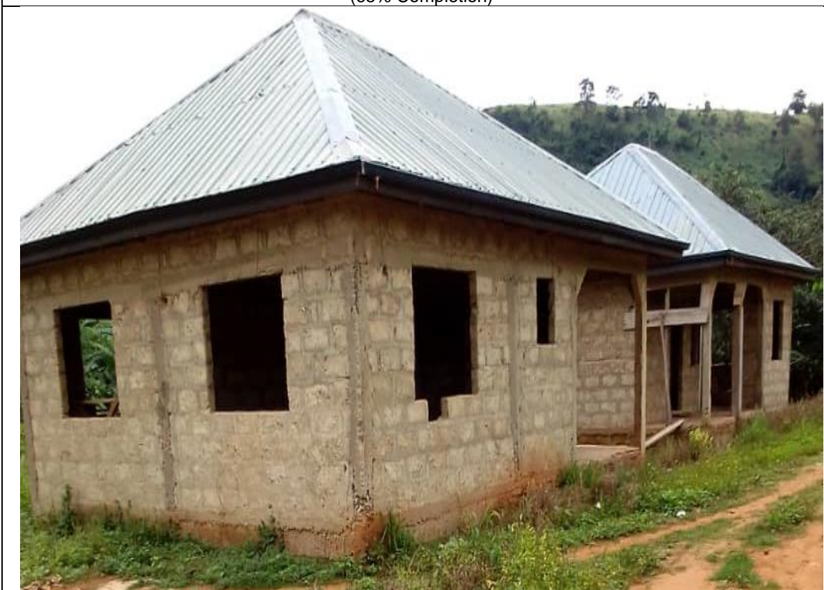
Completion of 1No. CHPS Compound with Out-House at Abisu
