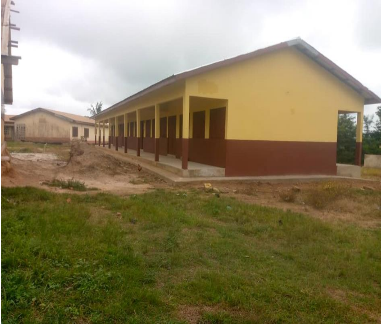
Construction of 1No. CHPS Compound with mechanized borehole at Atobriso currently at Roofing stage
