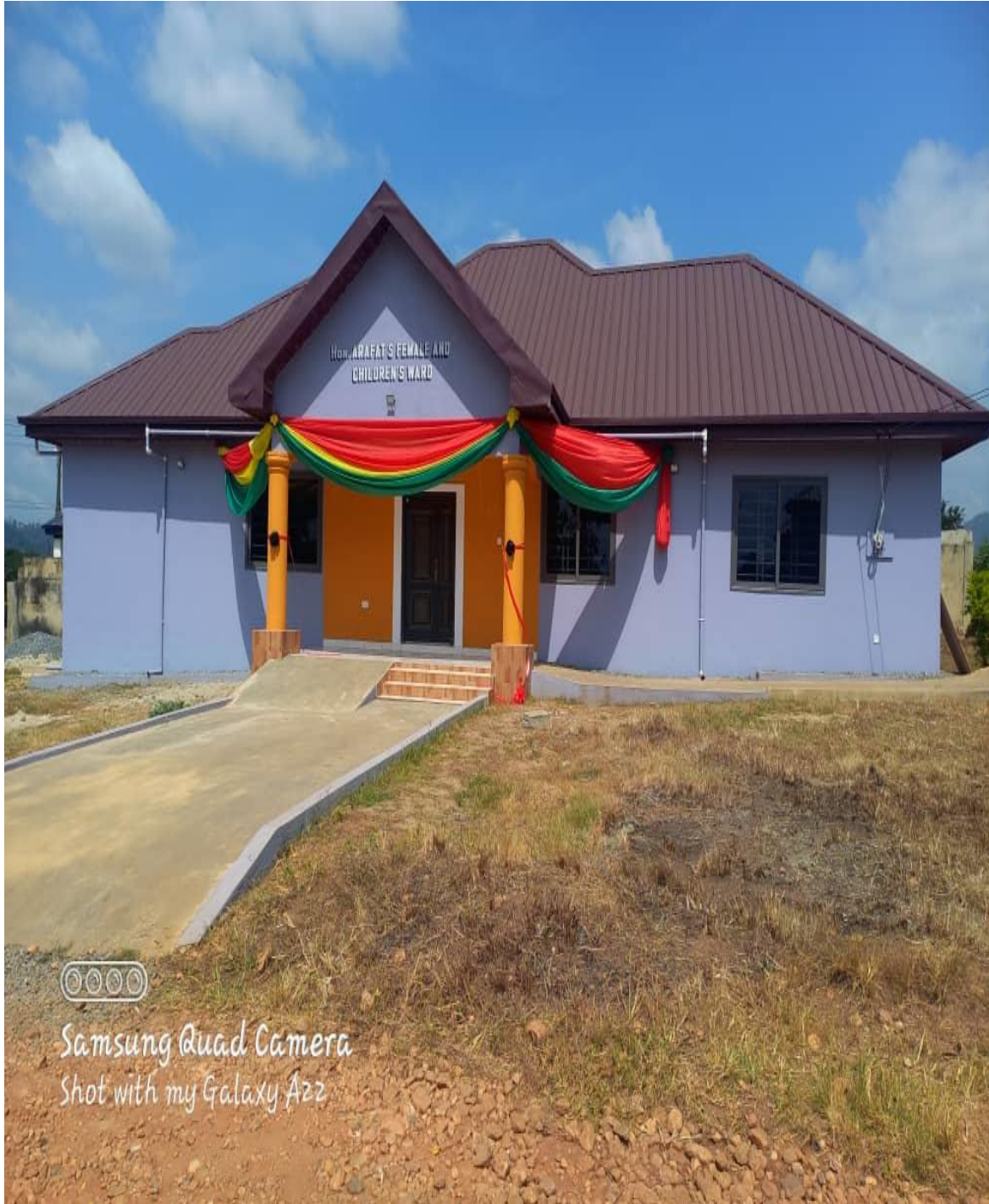
Constructed Female and Children's Ward at Osino Health Centre
