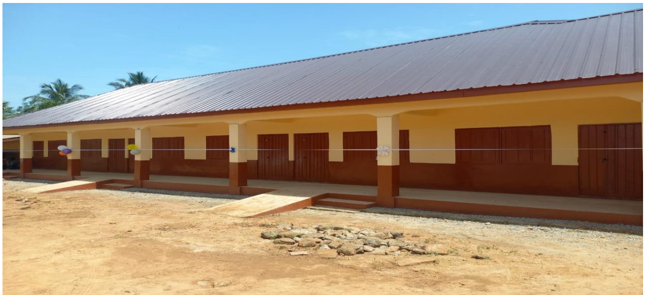
Constructed 3-Unit Classroom Block with ancillary Facilities at Akyem Nsutam Sda Jhs
