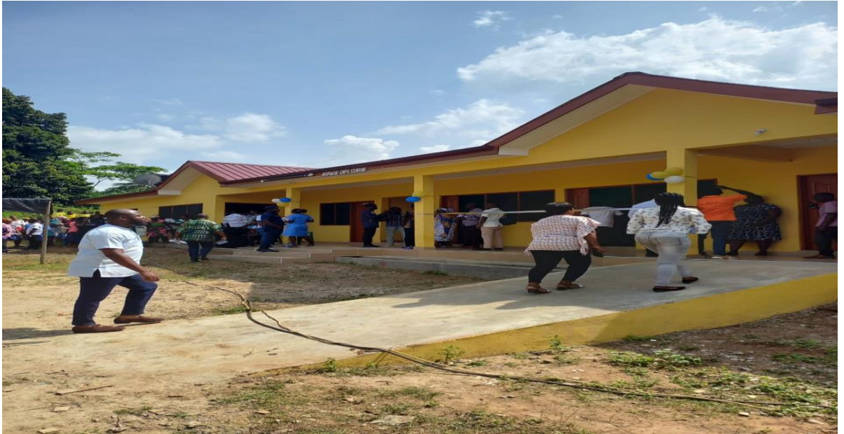
Constructed CHPS Compound and Nurses' Quarters at Bepose
