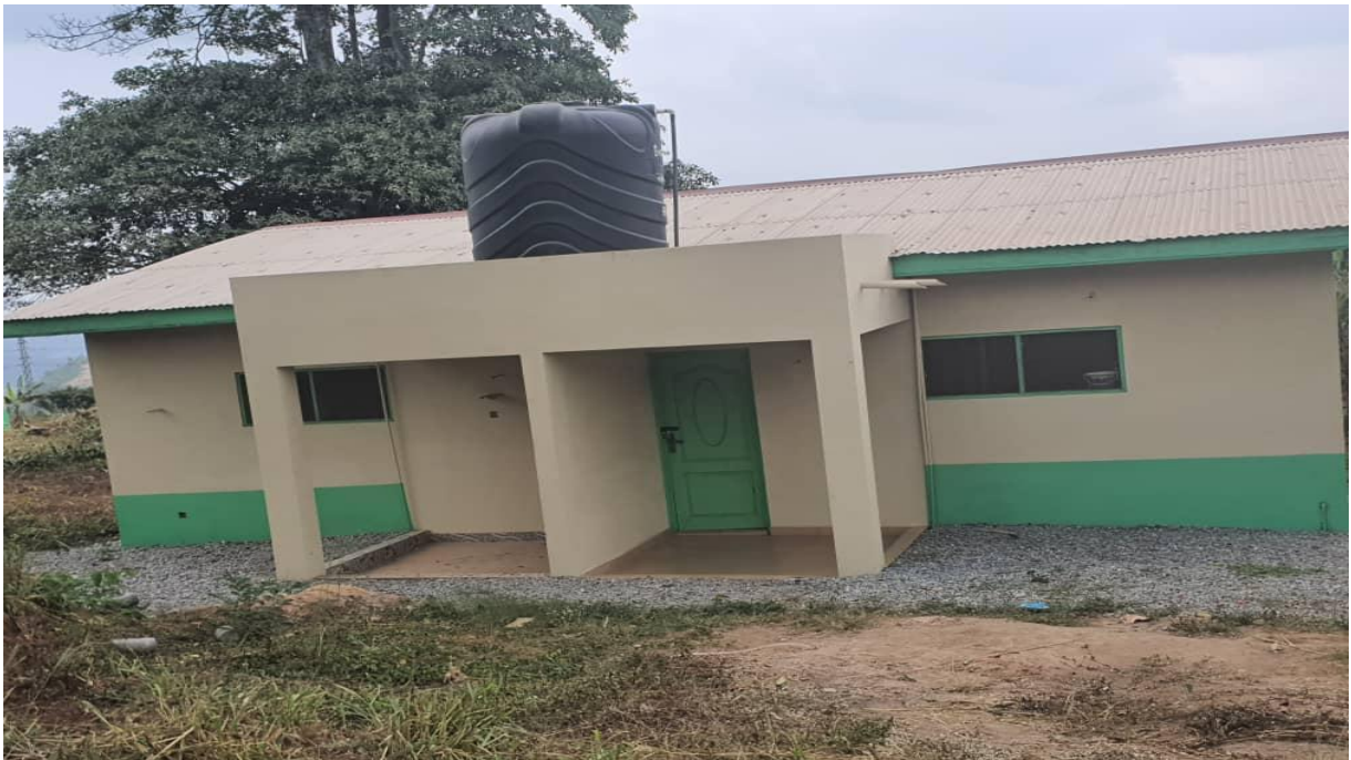
Achievement 5: Construction of 20-Seater W/C Toilet Facility-Adonten SHS
