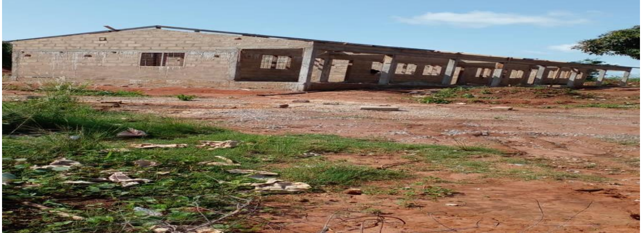
Figure 9: Completion of 1no. 3 unit CRB with ancillary facilities at Fawoman – DDF
