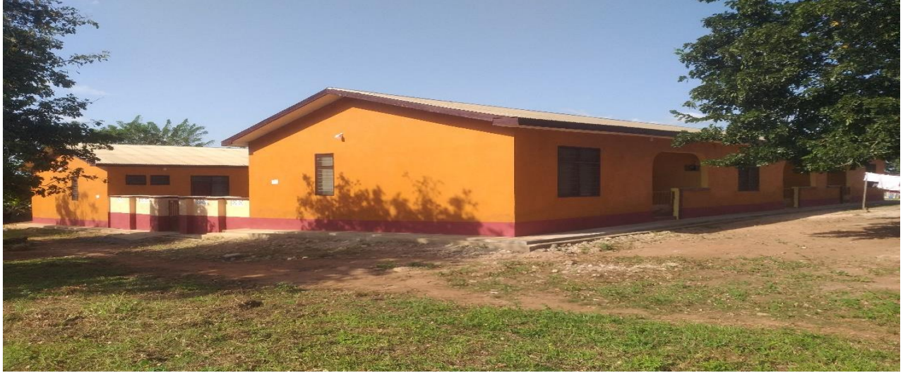
Figure 11: Renovated 1 no. 5 unit teacher's quarter at Beposo- DACF
