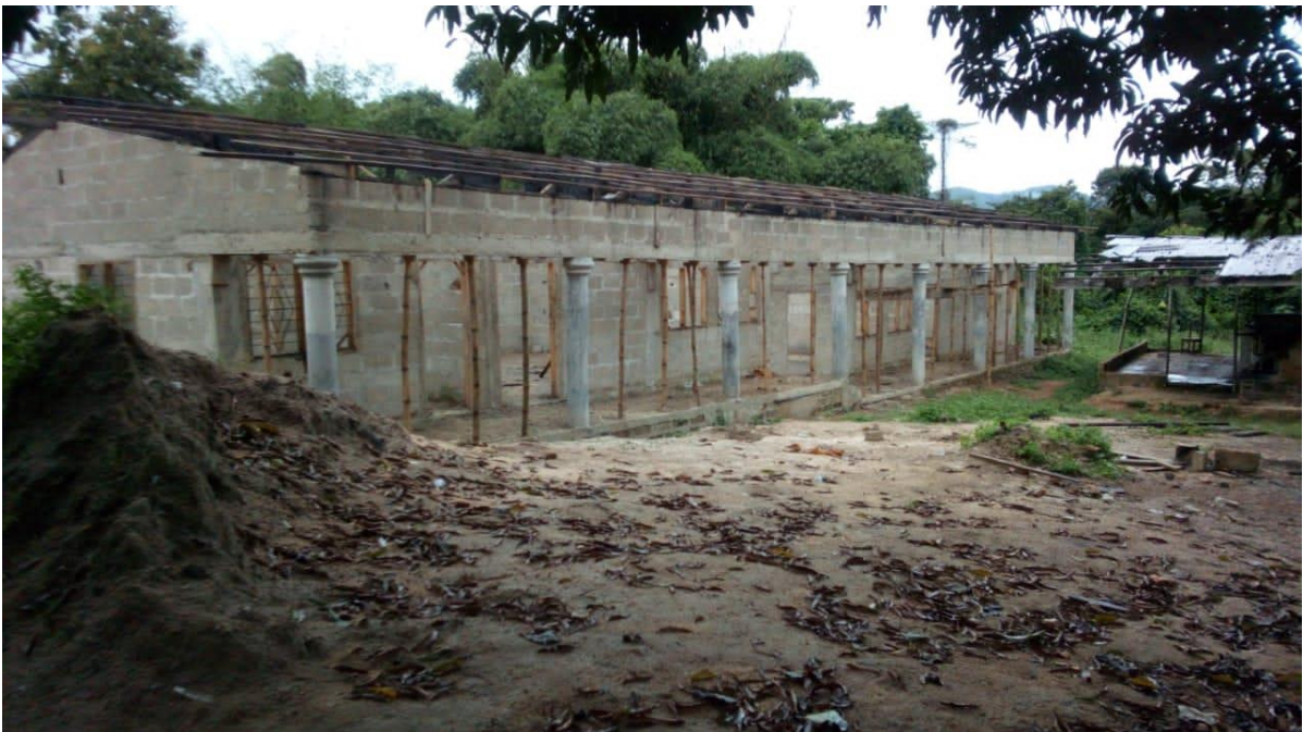
Figure 8: Construction of 1no. 3-unit classroom block at Adutwam – DDF
