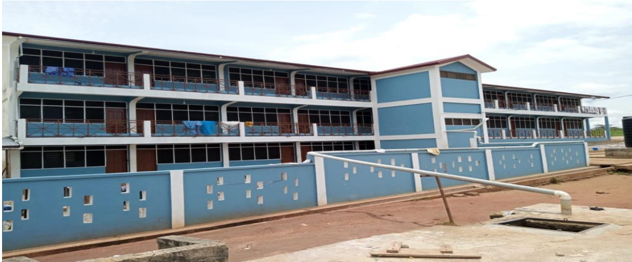
Figure 13: Complete the renovation of Nsutaman SHS Girls Dormitory block – DACF
