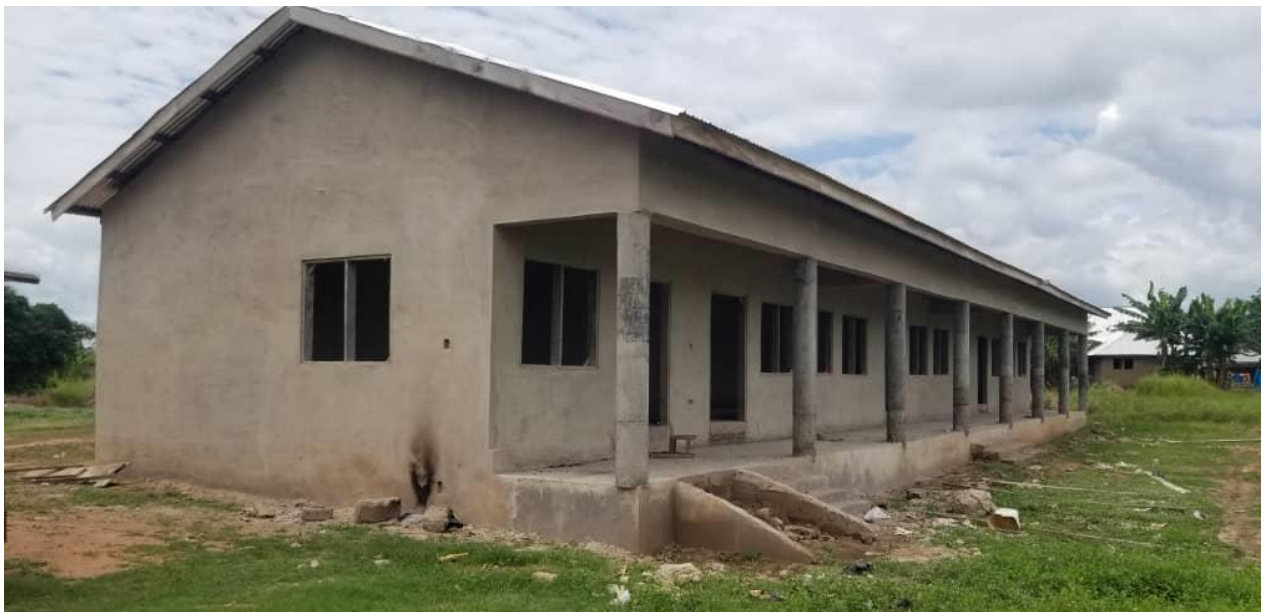
Figure 10: Completion of 1no. 3 unit CRB with Ancillary Facilities at Birem
