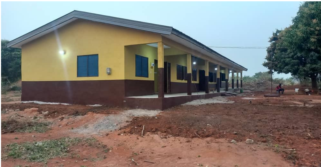
Figure 6: Completion of 1no. 3 unit CRB with ancillary facilities at Fawoman – DACF-RFG
