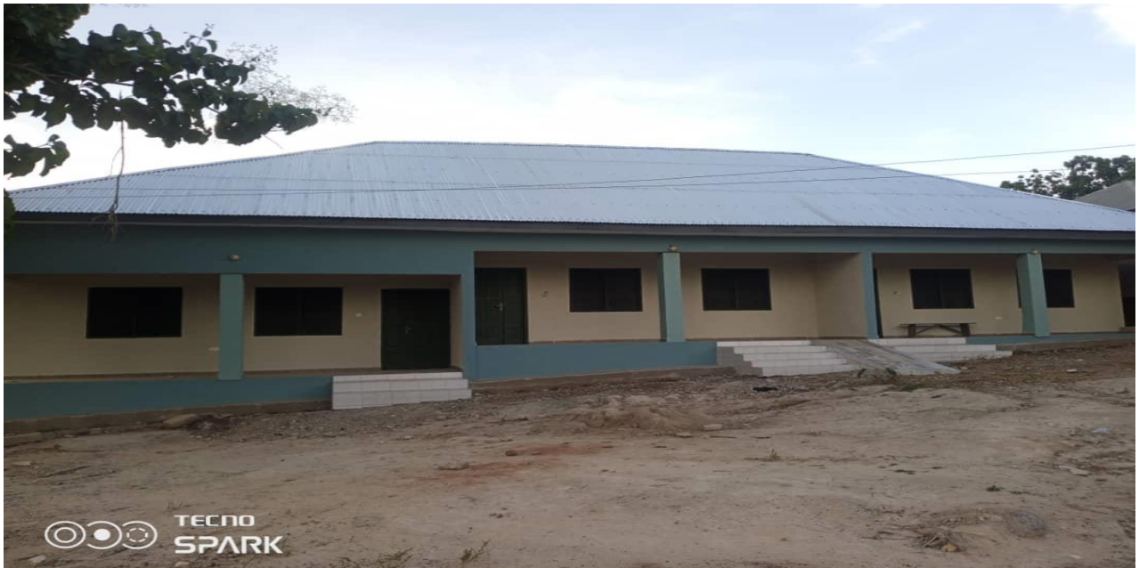
Figure 12: Construction of 1 no. 3 unit self-contained Nurses quarters at Beposo. –DDF
