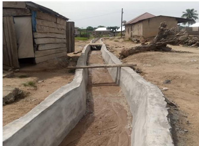
5. Construction of 400m U-Drain at Darso (UNCDF)
