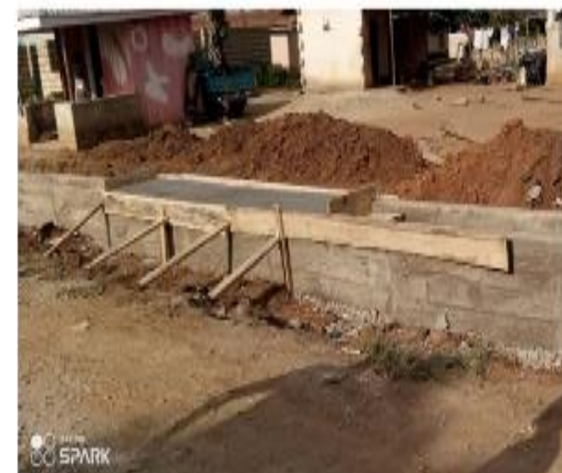
12. Construction of 3km u-drains in Akomadan-Kuneso (DACF)
