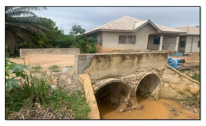
Constructed 8m Double 1800mm Diameter Pipe Culvert at New Nyamebekyere (MPCF)
