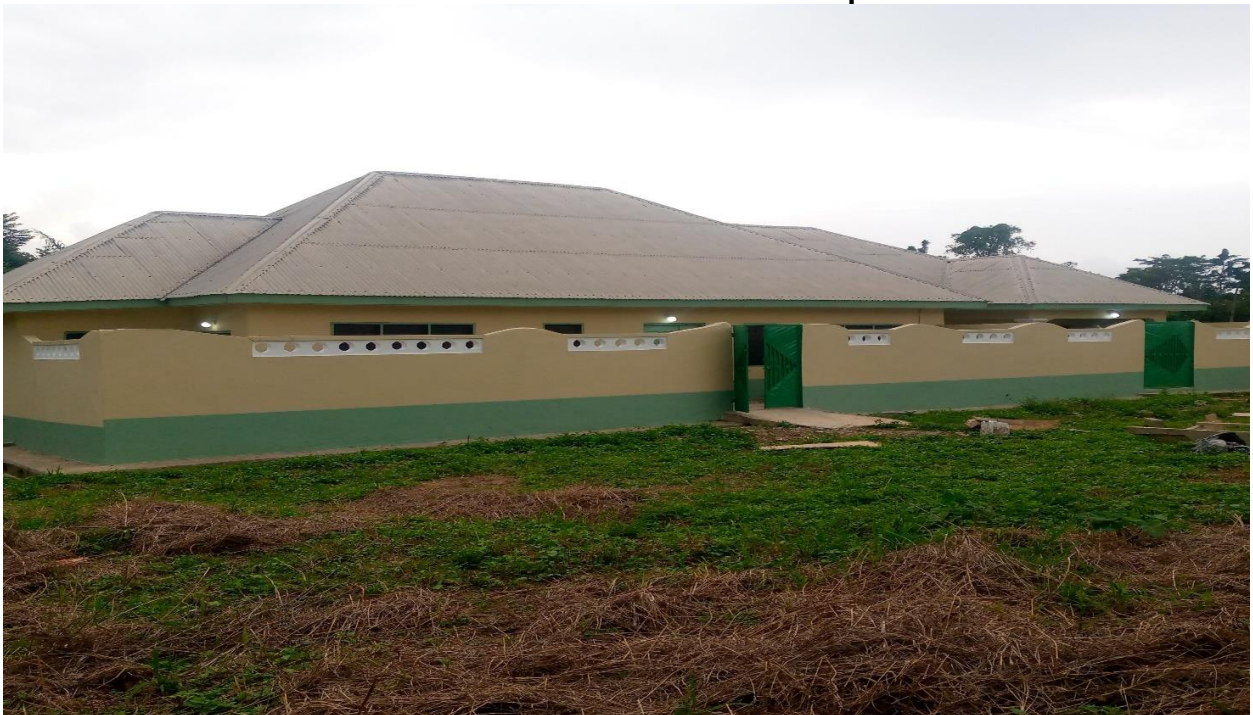
Renovated 1No. Bonkorkor CHPS compound
