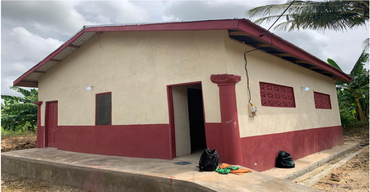
Completed 1No. 10-seater Aqua Privy at Essipong and Completed of 1No. 10-Seater Water Closet with 1No. Mechanised Borehole at Woarakose-DACF-RFG
