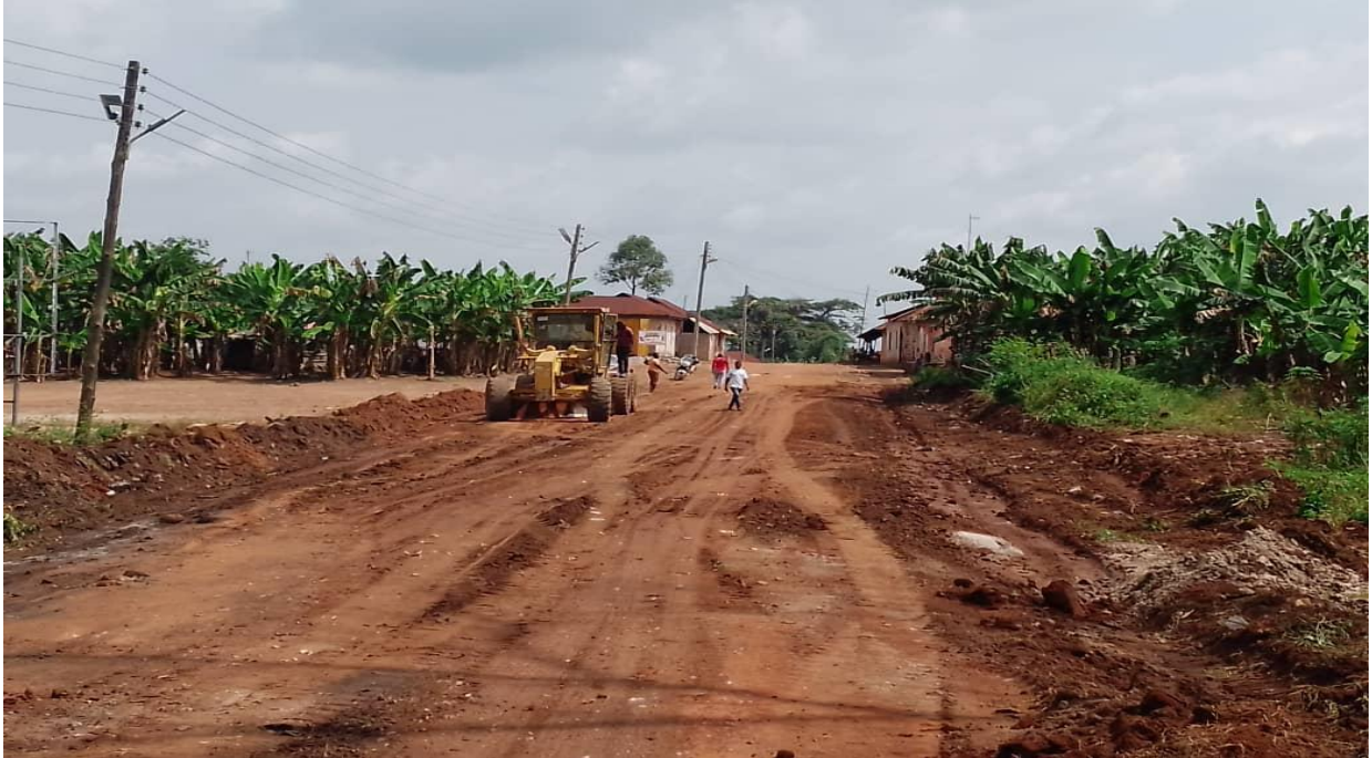
Reshaped 21.3km roads-DACF
