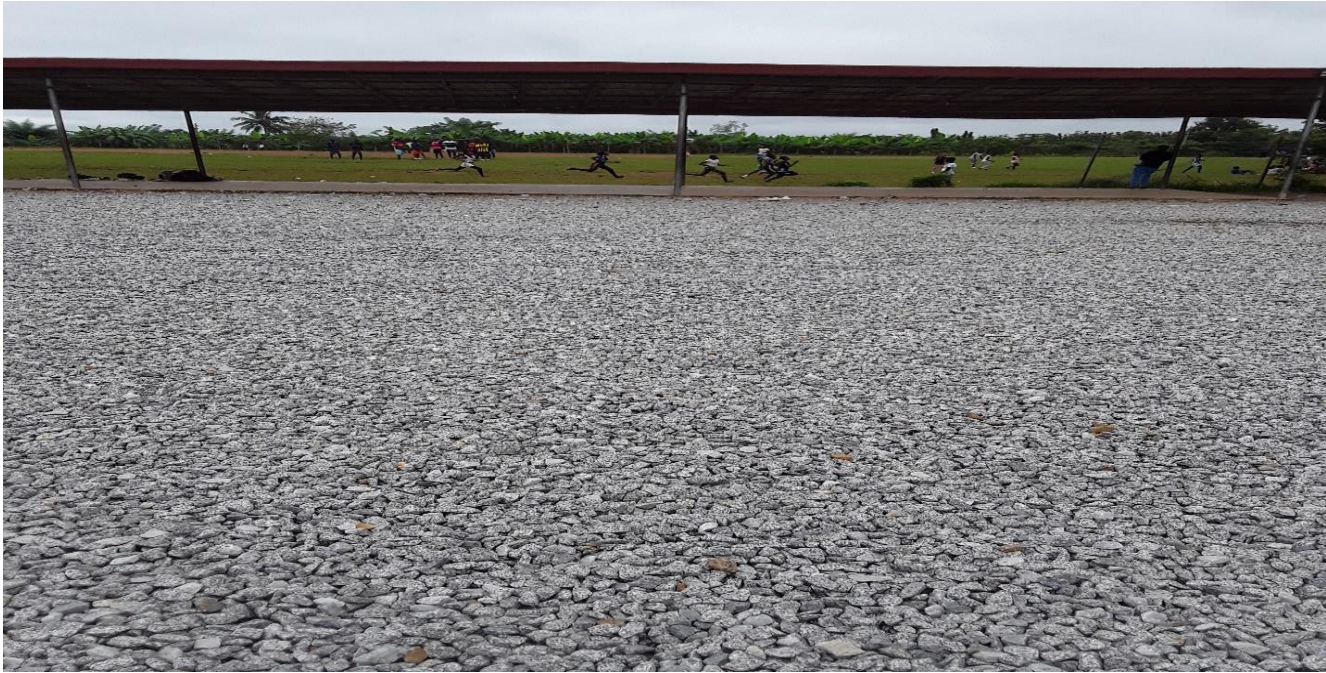
Constructed Lorry Park at Nkawie
