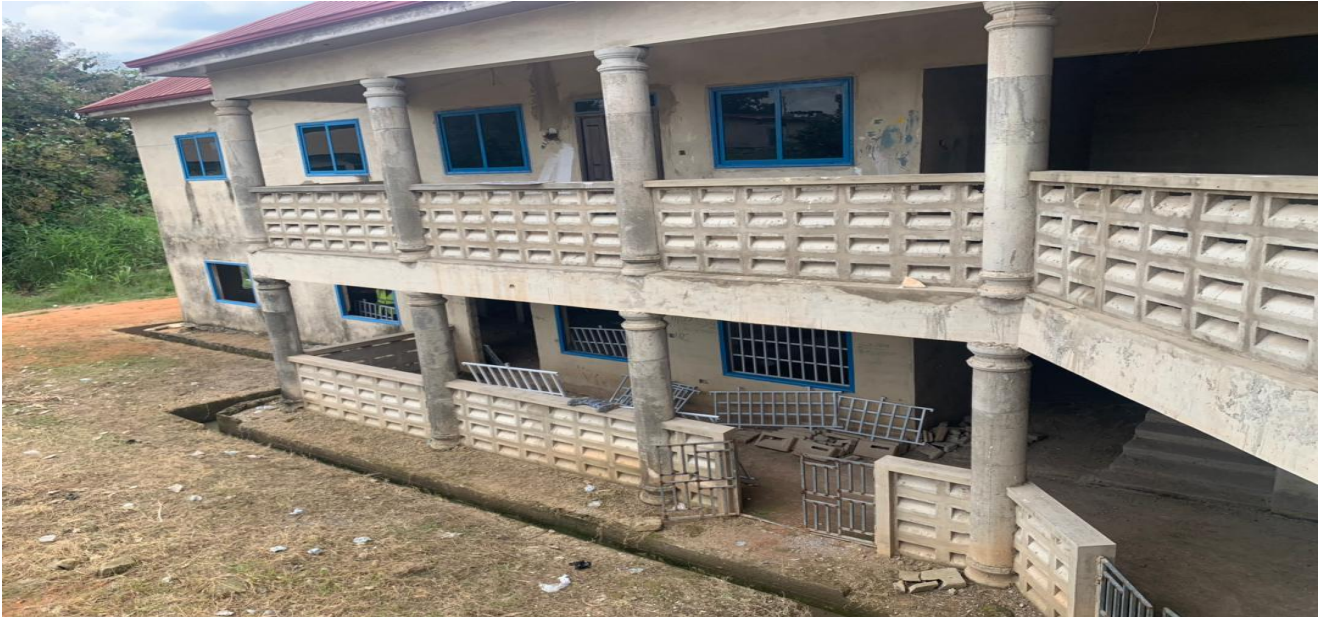
Completion of 1No. 1-Storey 6-Unit Flats at Toase
