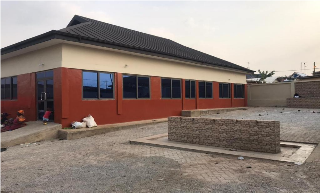
Completion of 1No. Meat Shop at Nkawie Market
