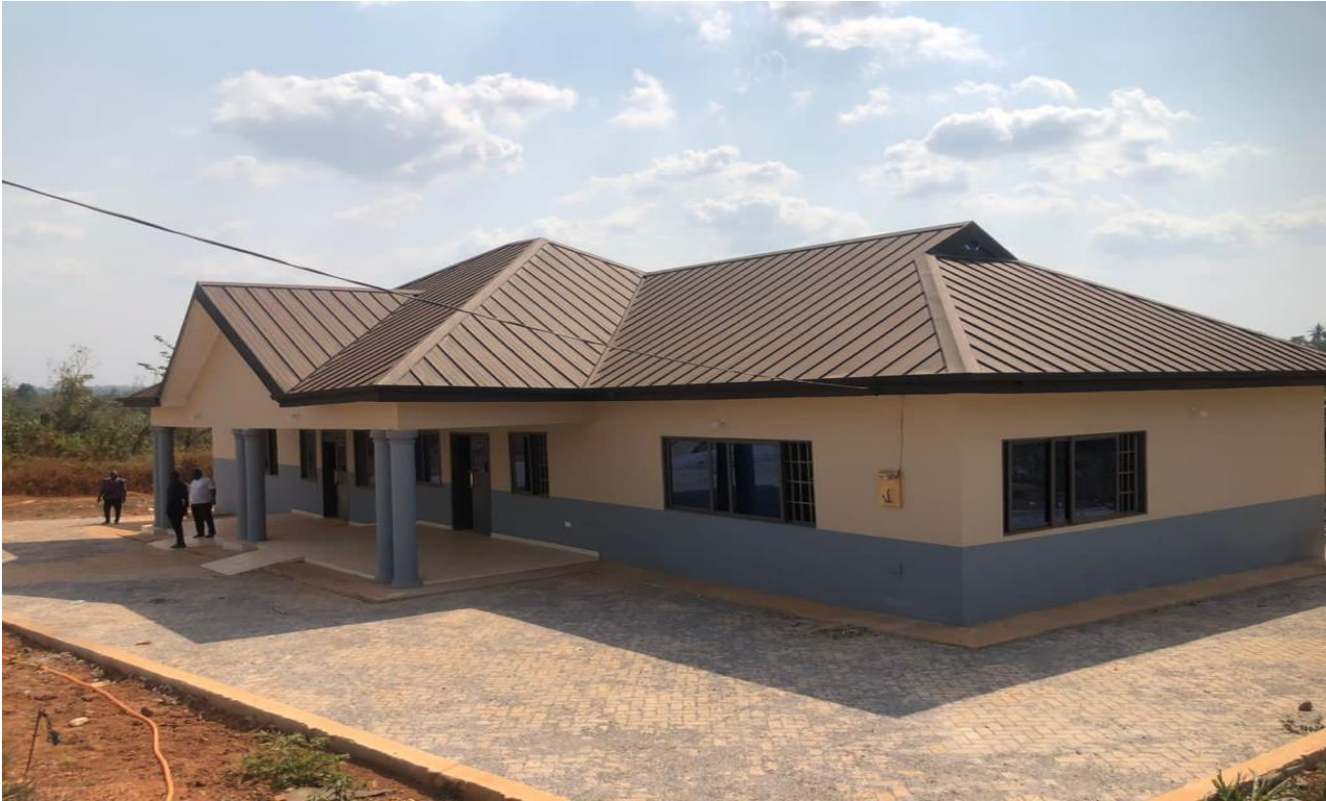
Constructed 30 Bed Capacity Ward at Asakraka
