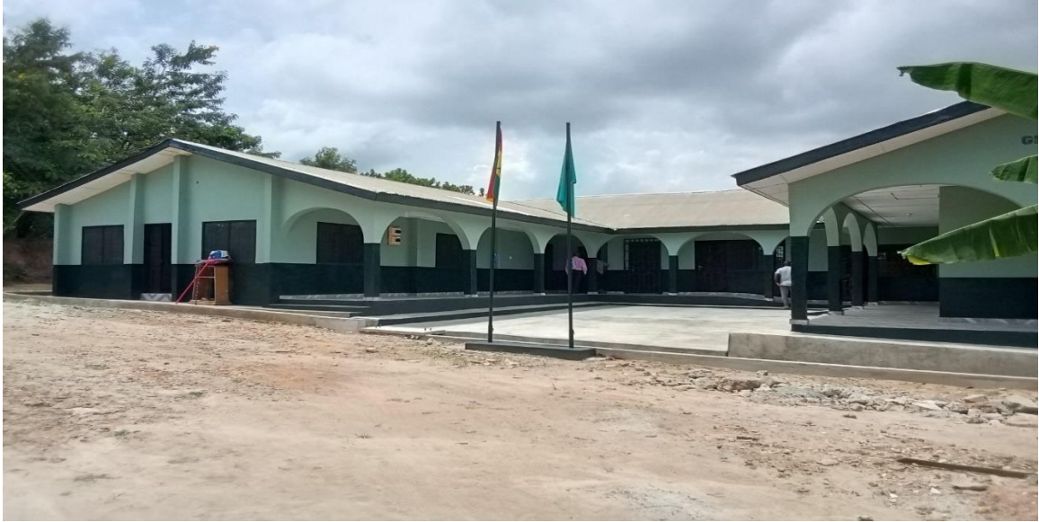
Figure 7: Area Council Office Renovated
